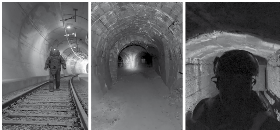
Figure 3: The Zentrum am Berg with different cross-sections and qualities of construction offers a perfect environment for research and development for subterranean operations from fully equipped road and railway tunnels via such similar to the London underground to narrow “Gaza Metro” style drifts. Pictures: Claudia Bendl (left) and author (middle, right).
